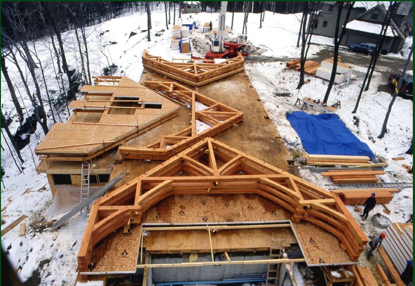
Breed Pool House Ready for Raising Douglas Fir Timber Hammer Beams with Arched Beams and Spar Urethane Finish Vermont Timber Works, Inc | vermonttimberworks.com
